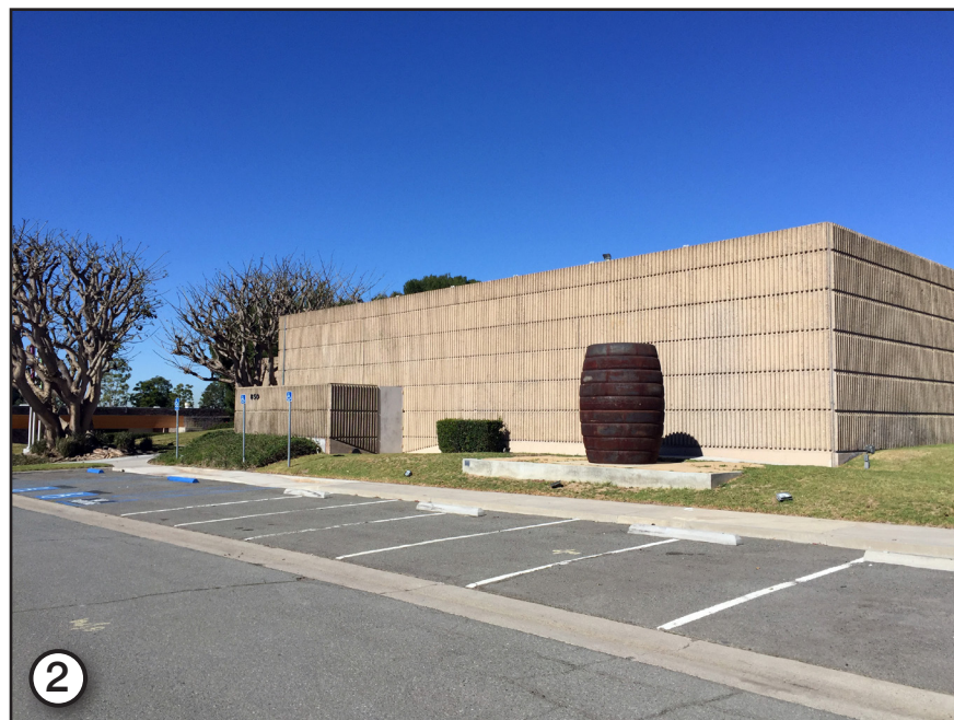
2 View of the southeastern building corner.
