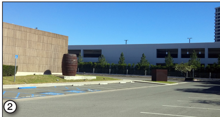
2 View of a multi-story parking garage east of the project site.
