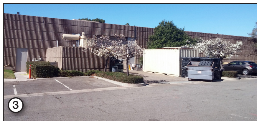
3 View of the eastern side entrance.
