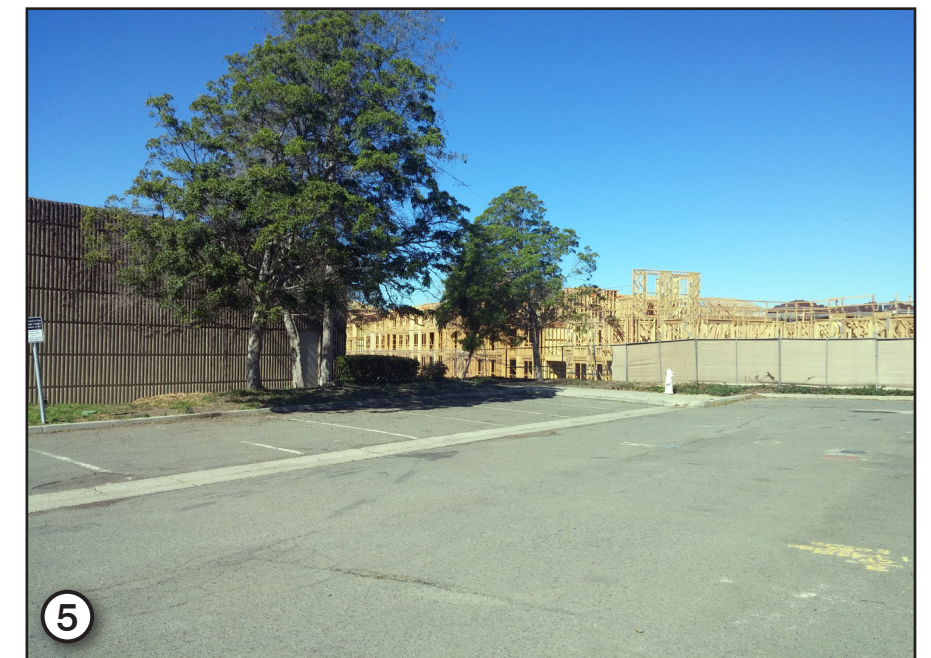
5 View of the northeastern building corner and adjacent San Joaquin Plaza residential construction.
