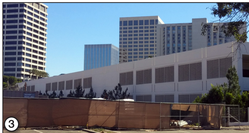
3 View of a multi-story parking garage east of the project site.
